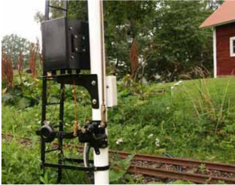
Figure 4: Close up of semaphore servo mechanism. The signal wing is connected to the counterweight arm, which in turn is lifted or lowered by a DC servo motor. The motor, its reduction gear and winding drum is housed in a watertight box and pulls the orange string. The rotation of the motor is controlled by end position microswitches. Microswitch responses and DC motor current are checked and controlled by the signal box computer via 4-pole electrical connection to the signal.
